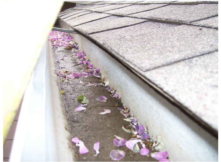
Clean the debris from gutters and downspouts and extensions
