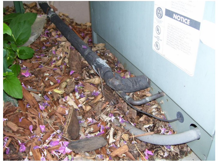
Repair the damaged A/C line insulation at the exterior unit.
