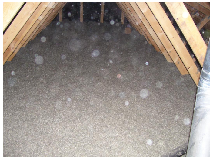
Well insulated attic space
