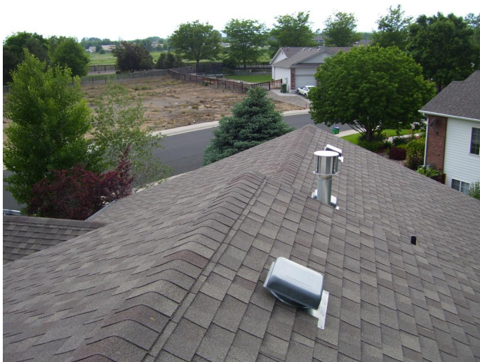
No missing shingles at this time
