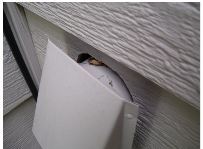
Seal all penetrations to prevent moisture/insect intrusion
